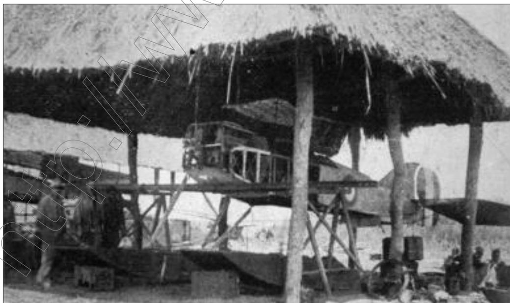
*This scene may show the repair of the second Short to be assembled, following its crash and recovery from the shallow waters of the Tongwe lagoon. Another machine stands with wings folded under its adjacent shelter, necessary to protect dope and fabric from the effects of strong sunlight. :Royal Military Museum, Brussels*
